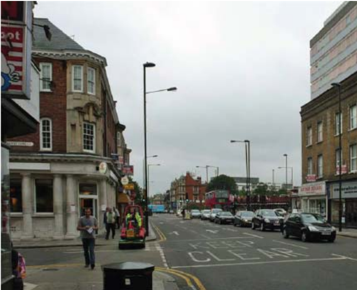
View south from Ballard's Lane of Existing Building
